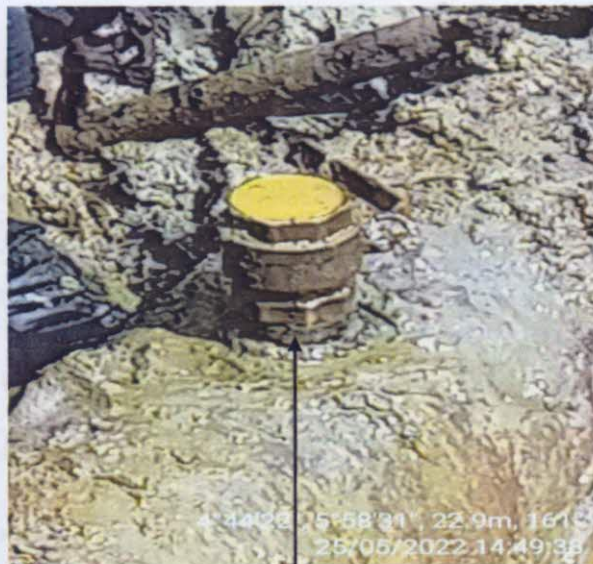
SPILL POINT (After excavation: Installed 3" valve at 12 O'clock position on the 14" pipeline)
